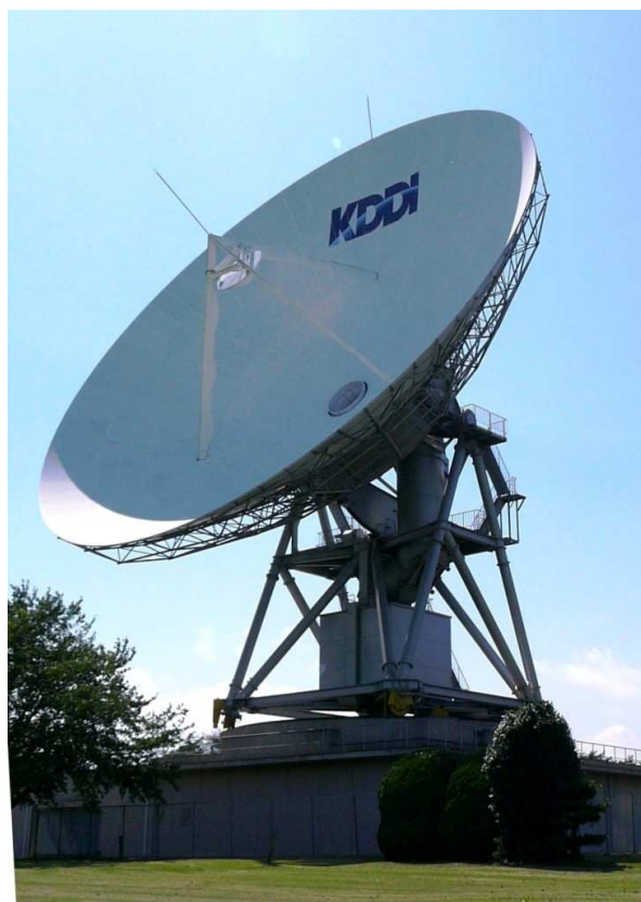
KDDI offered IBA-4 32-meter cassegrain reflecting dish was offered for radio amateurs' moon-bounce.
